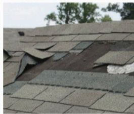
Missing Shingles
